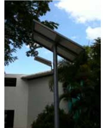
Street light equipped with Solar Panel (Sample)
